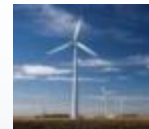
Clean Energy Storage
