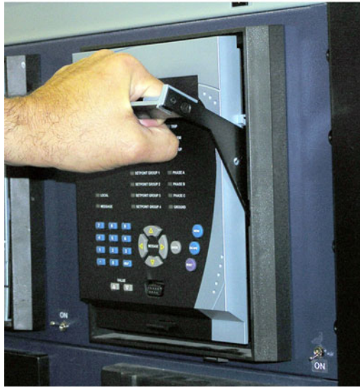
FIGURE 3-6: Rotate handle to stop position
