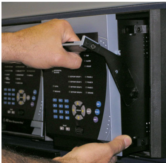
FIGURE 3-7: Slide unit out of case
