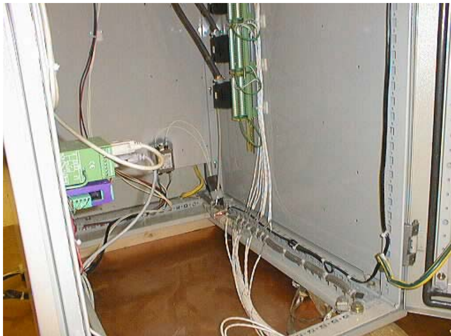
Figure 15-9—Bottom Cable Entry Area
