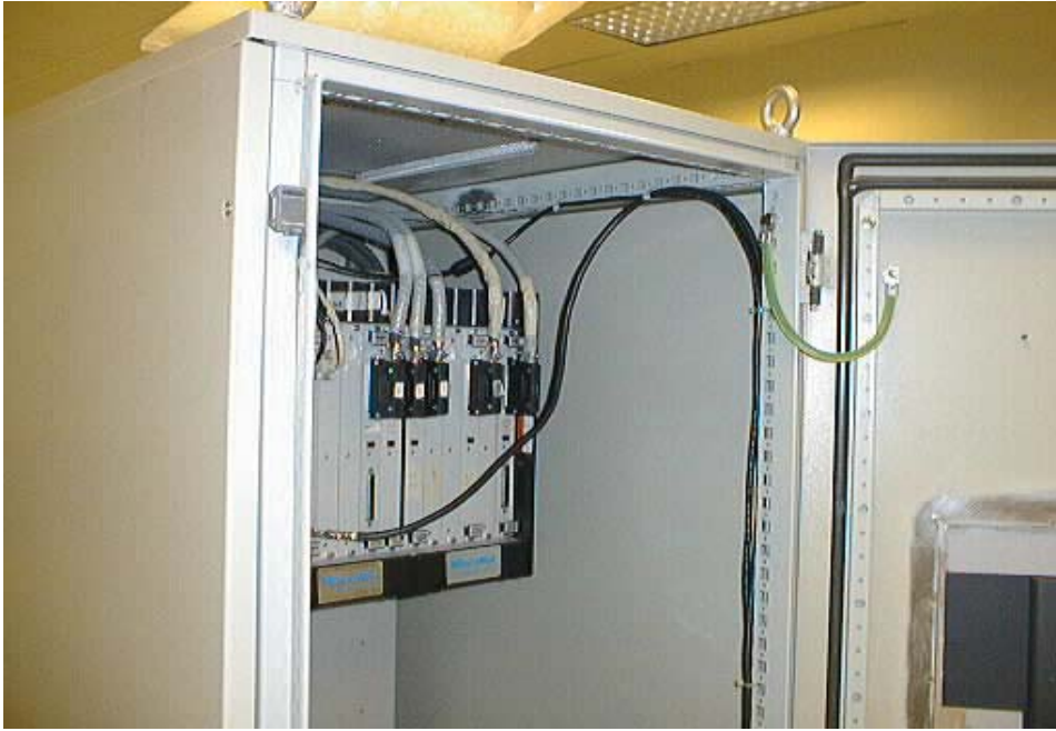
Figure 15-10—Door Bonding
